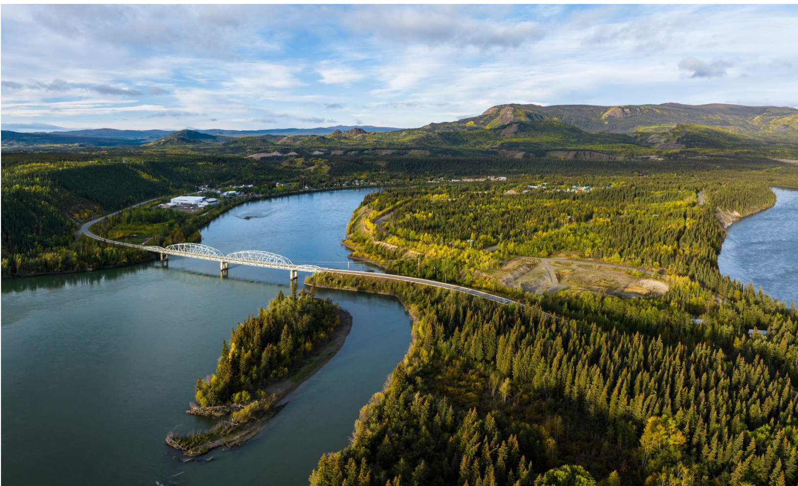
North Klondike Highway bridge over the Yukon River at Carmacks Photo credit: Government of Yukon / Andrew Strain
